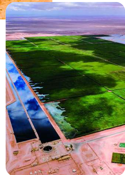
Aerial view of Nimr Oil Fields treatment wetlands
