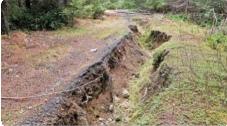
Removal of culverts on an unused road
