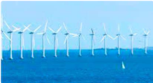
Wind turbines installed with use of ECONcrete 67
