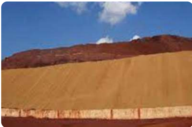
Operational iron ore mine with coir matting to reduce dust impacts and contribute to slope stabilization 38
