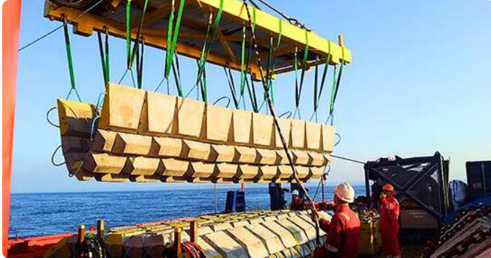
Roman Stone Construction Co. marine mattress being installed in the United Kingdom 75
