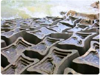
ECONcrete used in a coastal fortification structure 66
