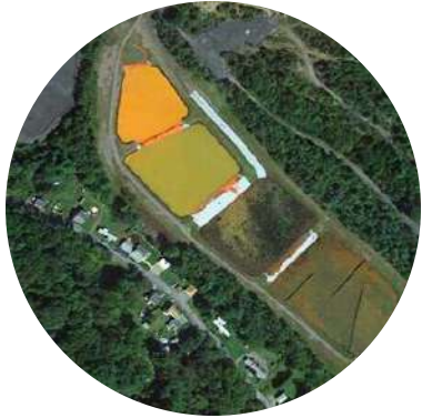
Silver Creek aerobic wetlands treatment system used to treat acid mine drainage in the United States 33
