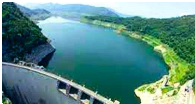
Reforestation surrounding Francisco Morazán Hydroelectric Power Station in Honduras 76
