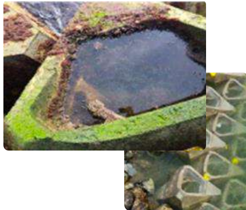
Pilot study of ECONcrete Coastalock armor units in the San Diego port 88
