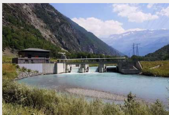
Romanche-Gavet, largest hydroelectric project in France Credit: EDF
